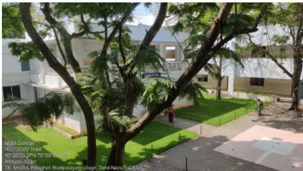
CONTROLLER OF EXAMINATION BUILDING
