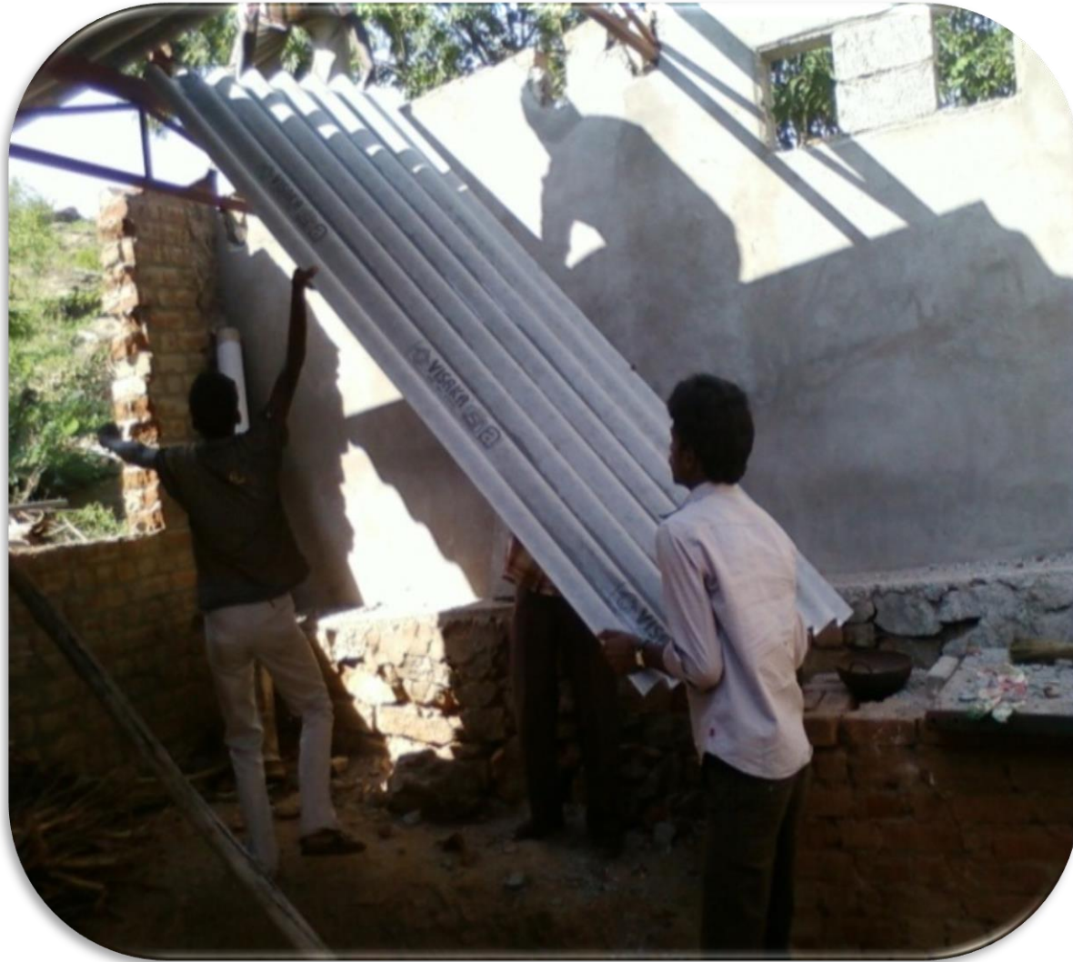
Kitchen Roof Construction on March 2013 at Child care Trust, Thali
