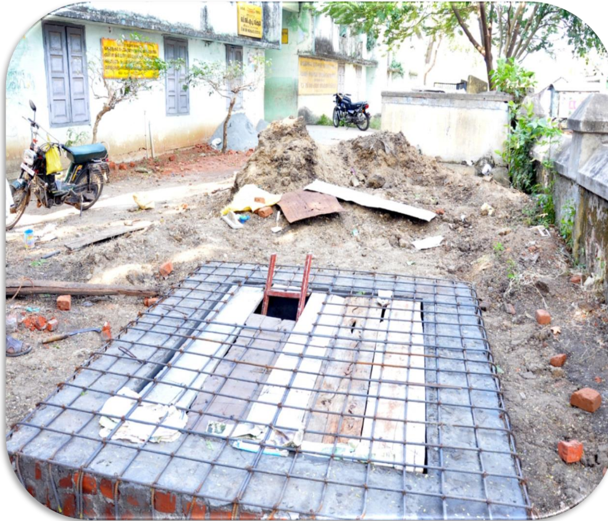
School water tank contribution by our students to Government School, Vannamadai December 2012
